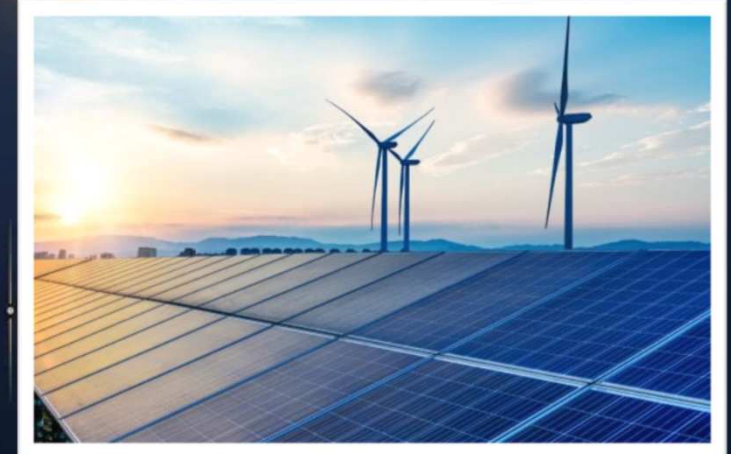
Renewable Energy Plant
